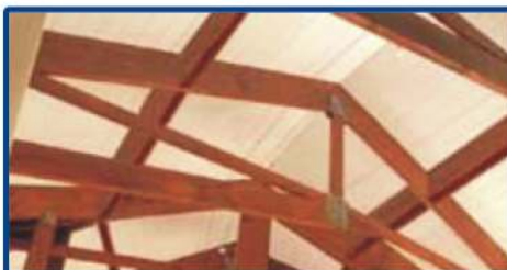
Used over beams as an internal ceiling and insulator
